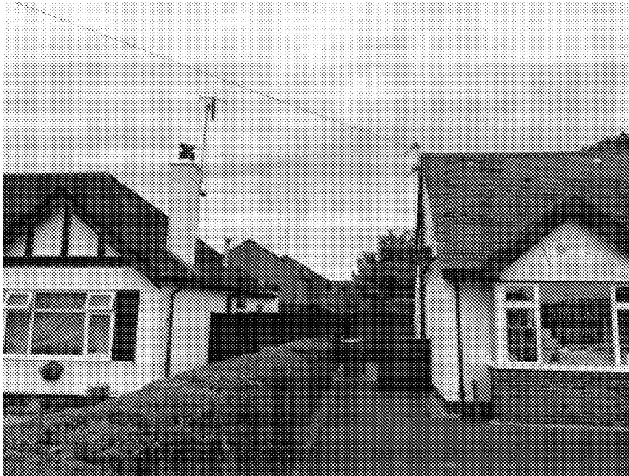
Photograph 02 - Showing the side access to the rear of the house
