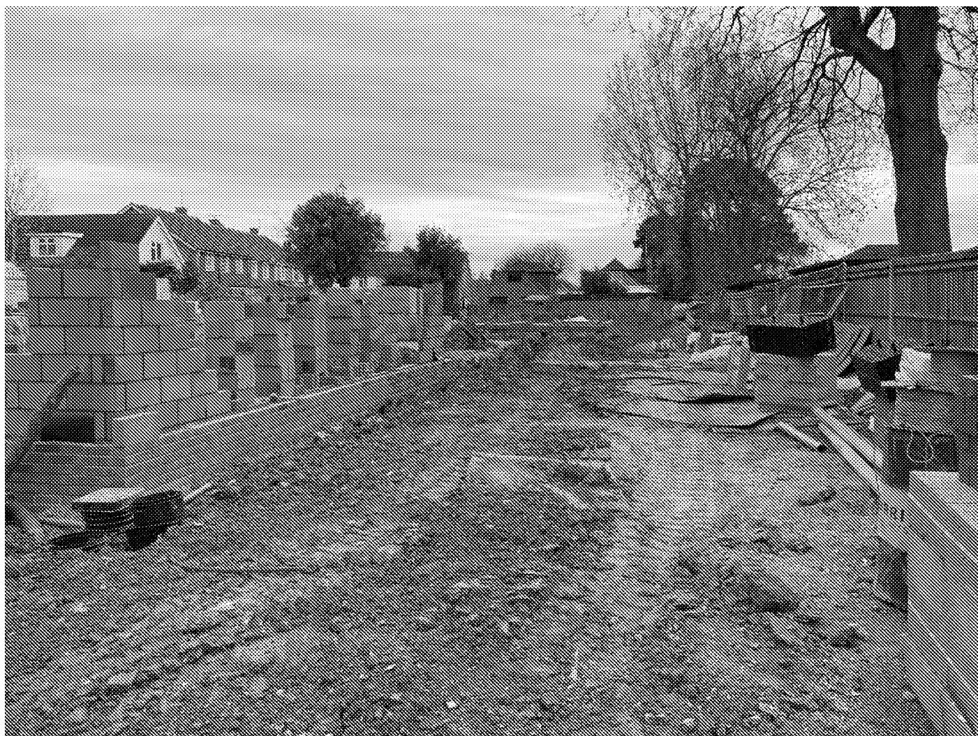
Fig.3. Looking south from near entrance to site, showing progress of above ground construction.
