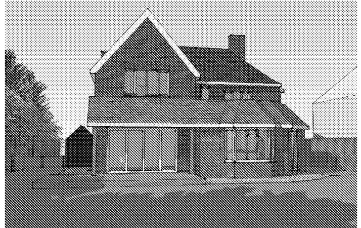
Comparative view to show how the existing single-storey roofline is continued to form a covered veranda
