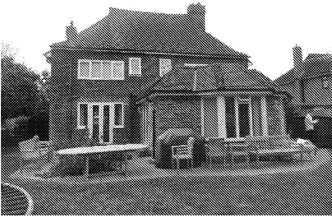
Comparative view to show how the existing single-storey roofline is continued to form a covered veranda
