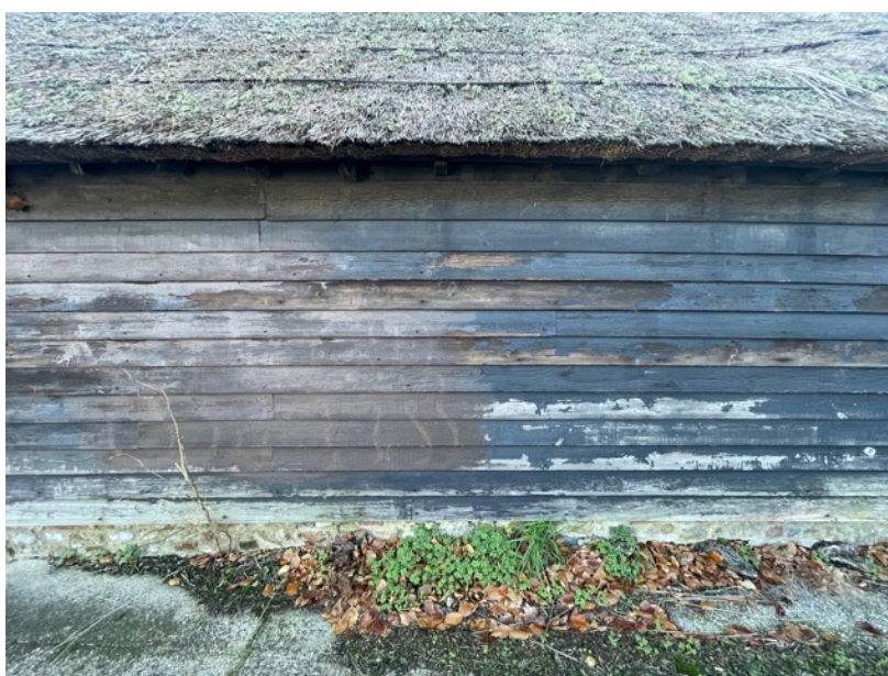
fig 9-10 Existing timber frame wall / weatherboarding.
