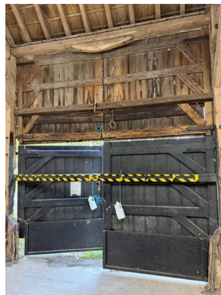
fig 14 Existing barn doors (SE elevation)
