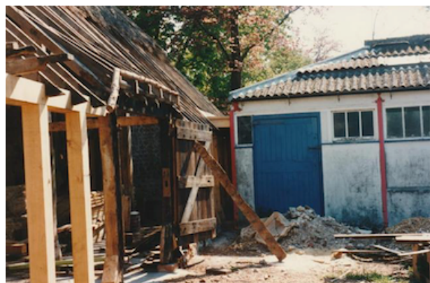
fig 7-8 Previous replacement of rear timber frame wall.
