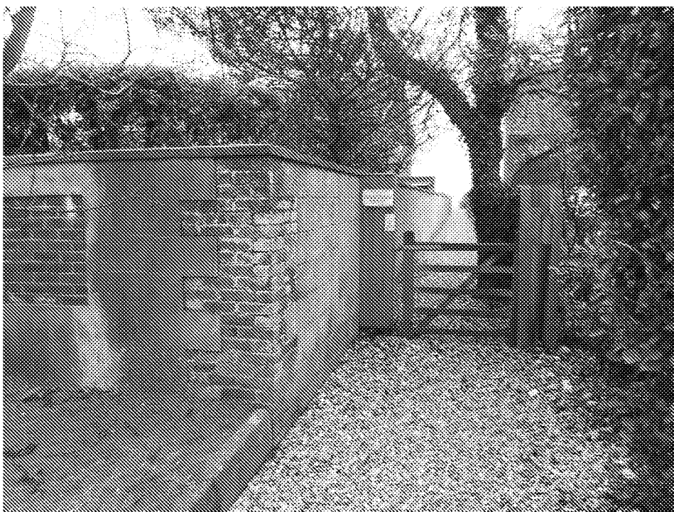
1.4 – Public foot path [access to beach] along west boundary
