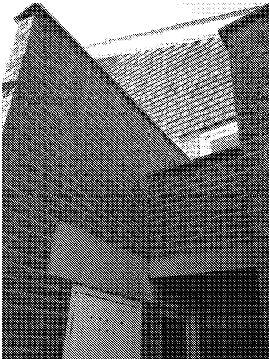
1.11 – Existing terrace [west elevation]
