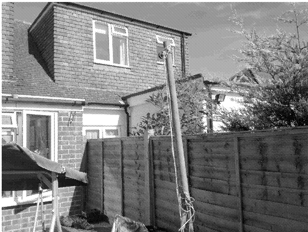
View looking towards rear elevations of 35 & 37 Lincoln Av. This shows bedroom window of 35 along with existing rear extensions to both properties. Recent planting by neighbour is also clearly evident.
