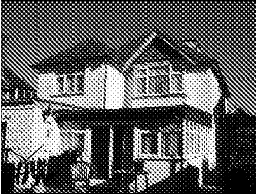
Photograph 1. Showing the west elevation of Building A.
