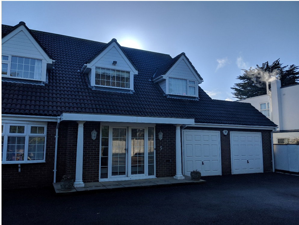
Fig 2. View of house from north (driveway)
