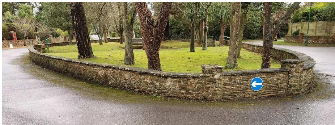
13 – Fairway roundabout – stonework
