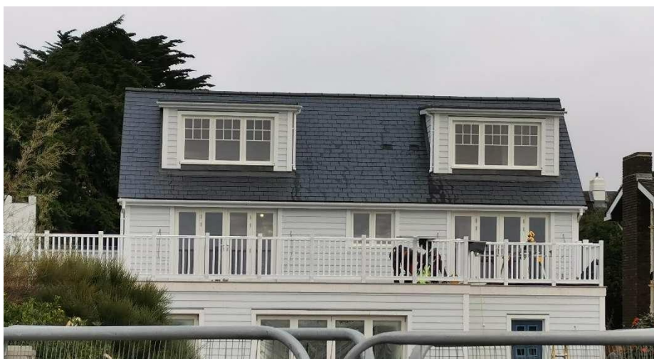
10 – Property under construction Bay Walk – Boarding & Slate
