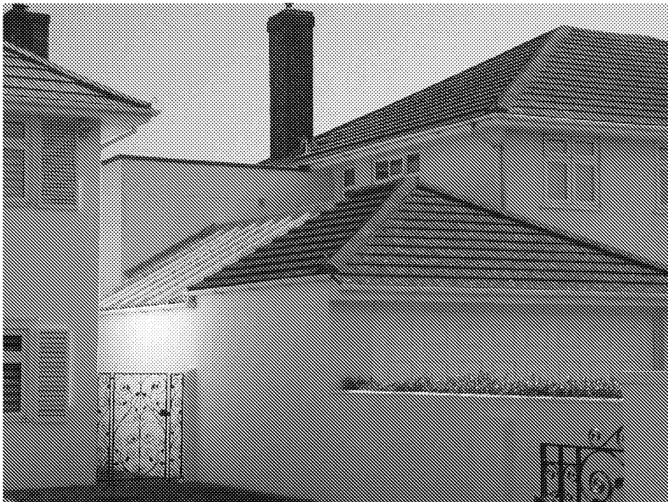
Picture – The existing flat roofed annexe extension and garage to the front.
