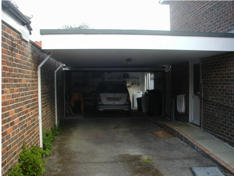
Picture – Car port and garage as exists.
