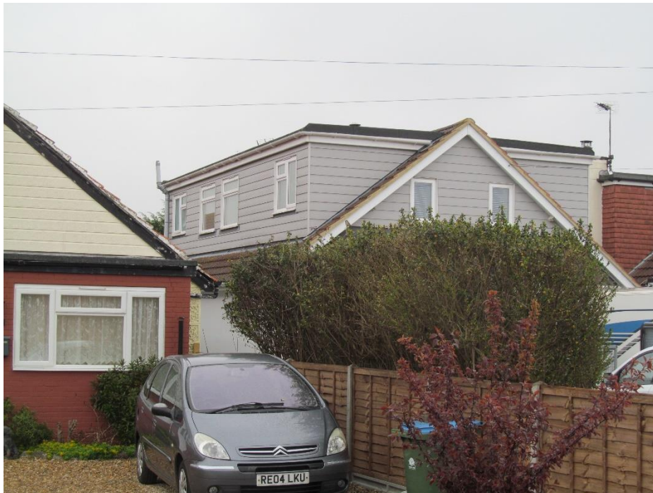
Front View No 114 Rose green Road. Similar larger extension
