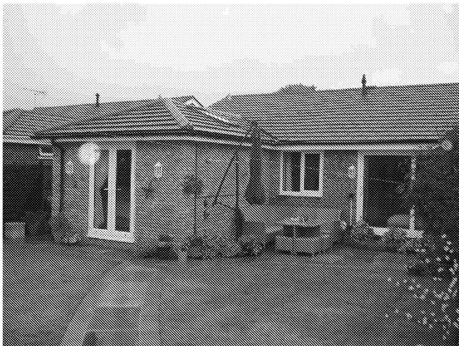
Photo 1 to show: House rear elevation – existing
