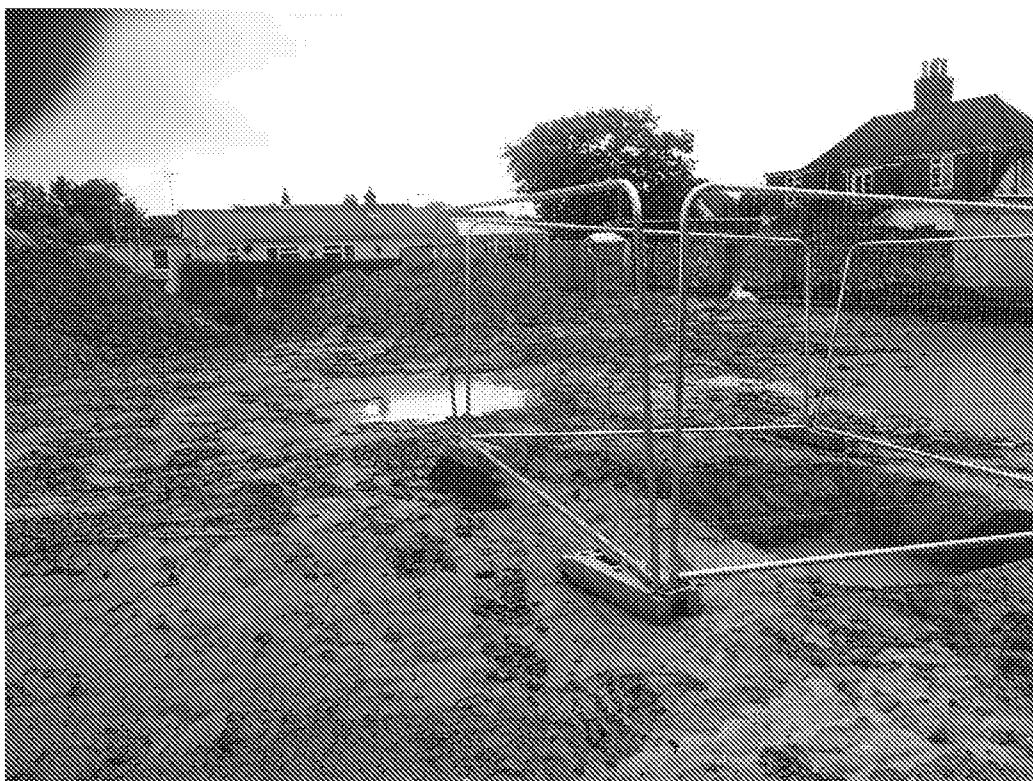
Photograph 17: General view across the site towards the south east corner of the site, foreground shows former manhole/cess pit excavated – 3 August 2017
