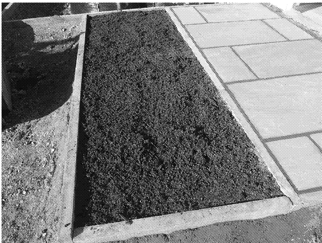
Photograph 25: General view of topsoil placed to front garden plot 1 – 20 February 2019
