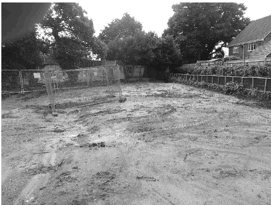
Photograph 14: General view of south west corner after completion of the made ground scrape – 3 August 2017
