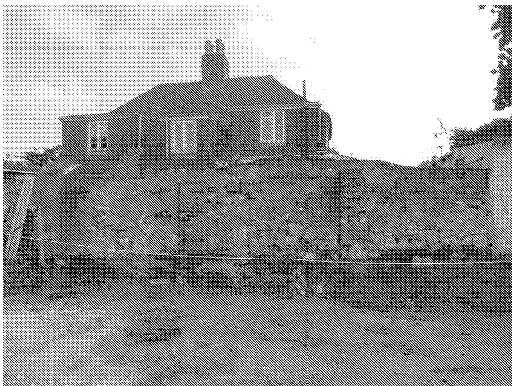
Photograph 12: General view of south boundary wall – 25 July 2017
