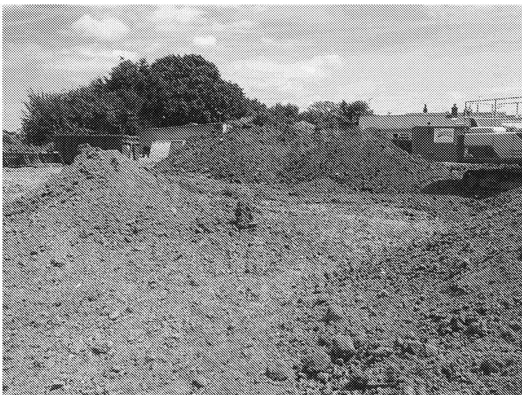
Photograph 7: General view of made ground stockpile – 17 July 2017
