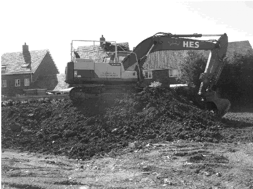
Photograph 3: Excavator stockpiling made ground material from the north side of the site — 13 July 2017
