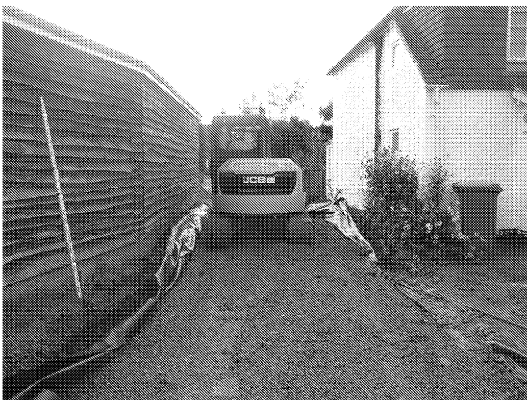
Photograph 18: General view of access lane with made ground replaced with crushed rock on a geotextile – 3 August 2017
