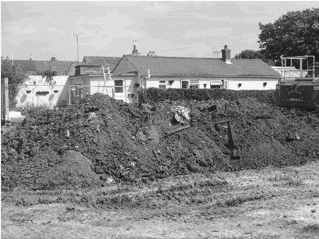
Photograph 10: General view of made ground stockpile towards the east of the site – 25 July 2017
