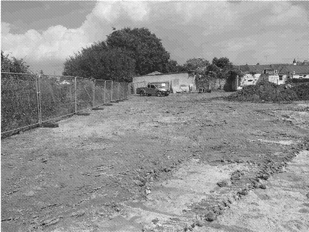
Photograph 9: General view of final scrape along the north boundary of the site – 25 July 2017
