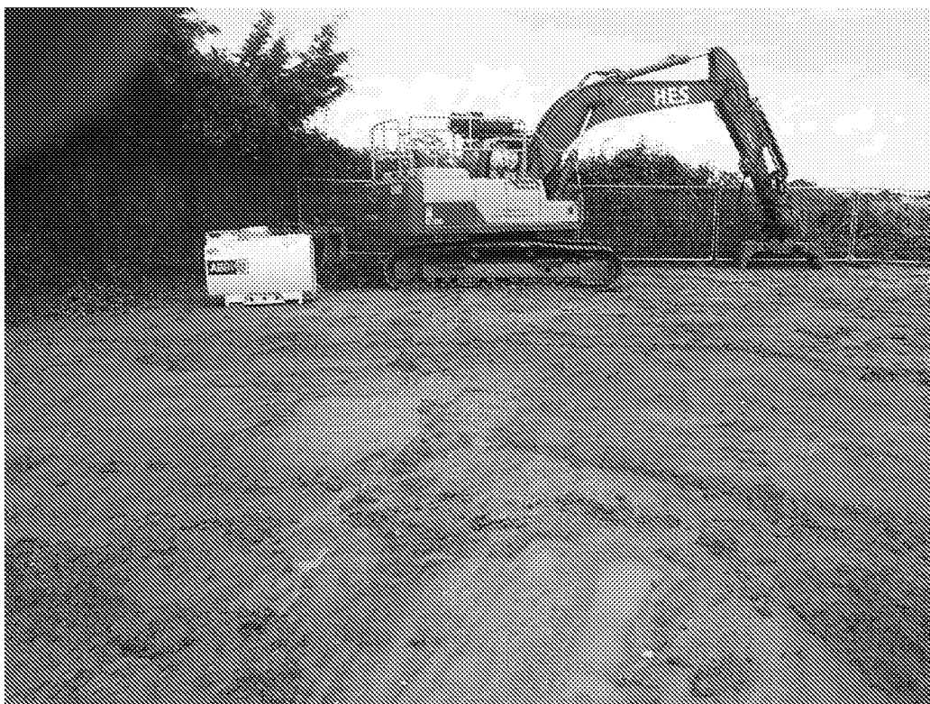
Photograph 15: General view of north west corner after completion of the made ground scrape – 3 August 2017
