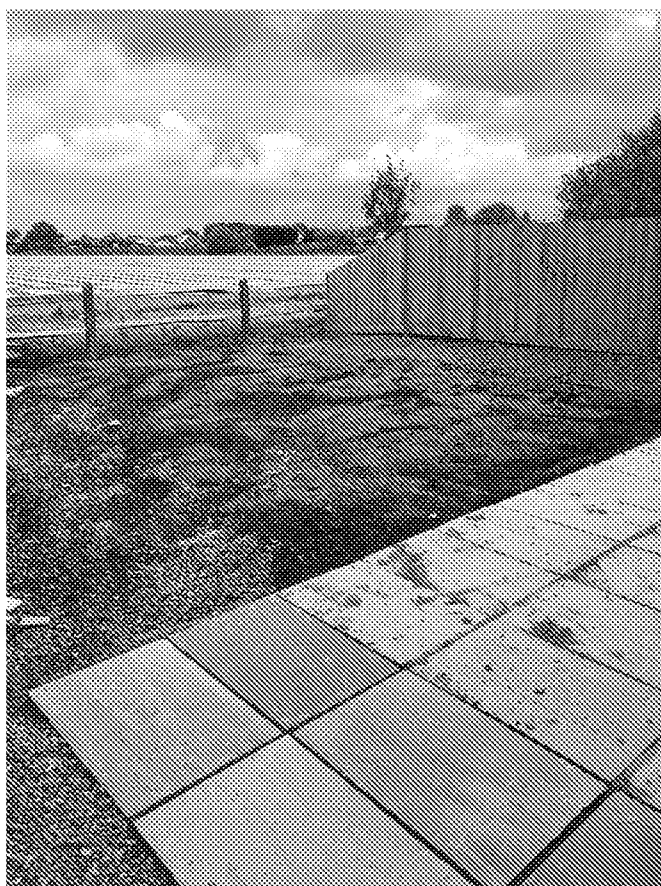
Photograph 35: General view of topsoil placed in plot 4 rear garden – 9 May 2019
