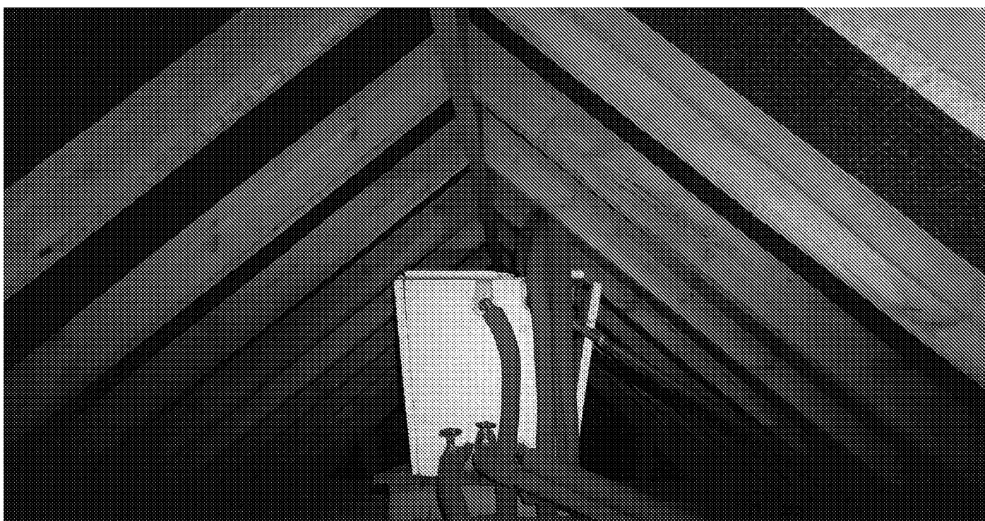
Photograph No. 6 - Internal view of Building No. 01: No evidence of bat usage was recorded within this building.
