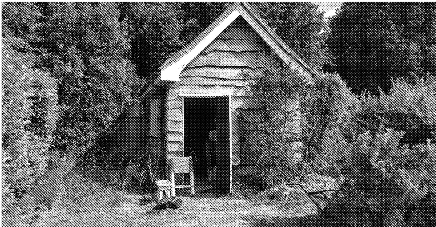
Photograph No. 3 - Building No. 02: No evidence of bats was recorded anywhere within this building.
