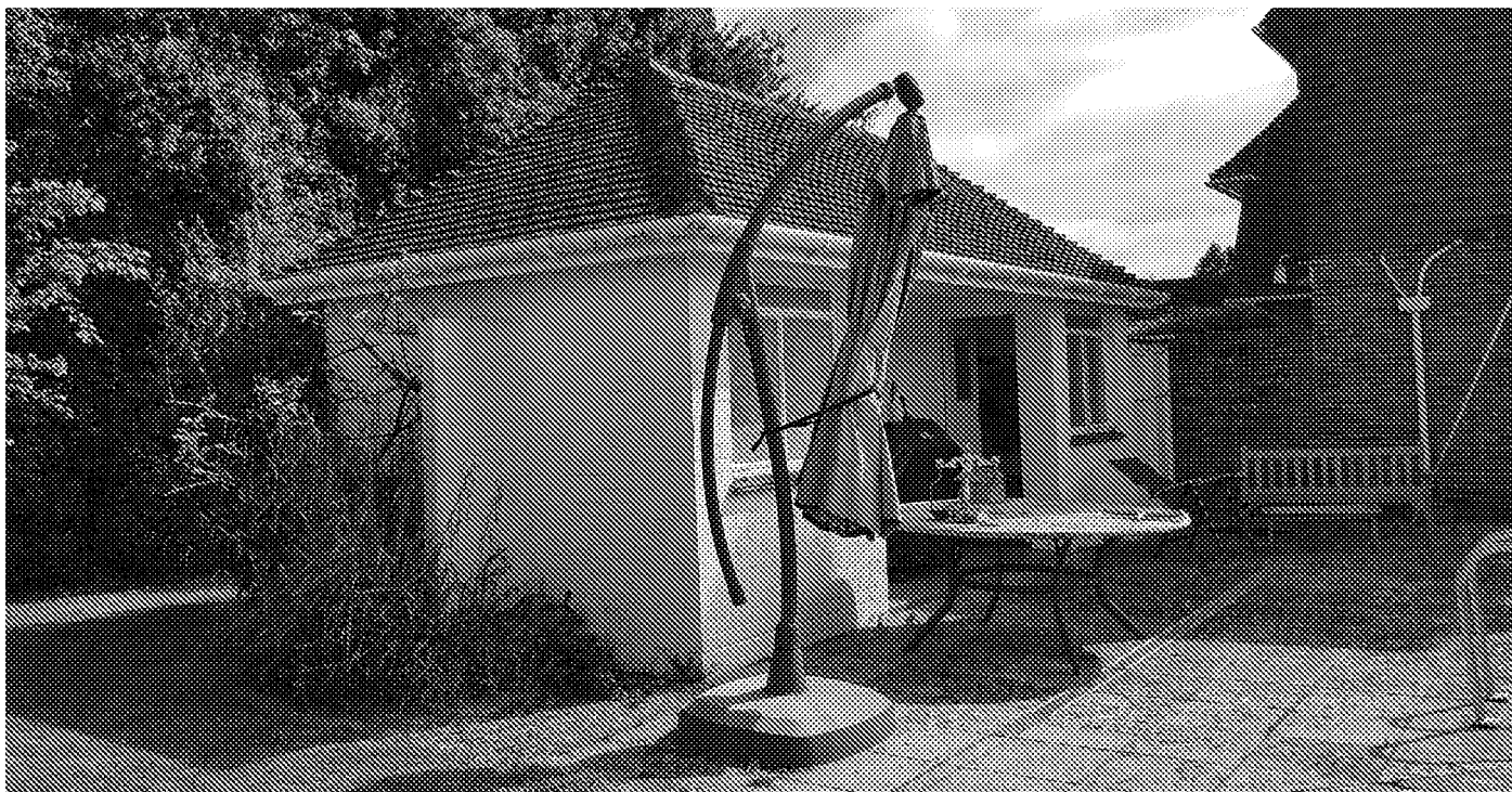
Photograph No. 5 - External view of Building No. 01; the building is considered to offer 'negligible' bat roost suitability.
