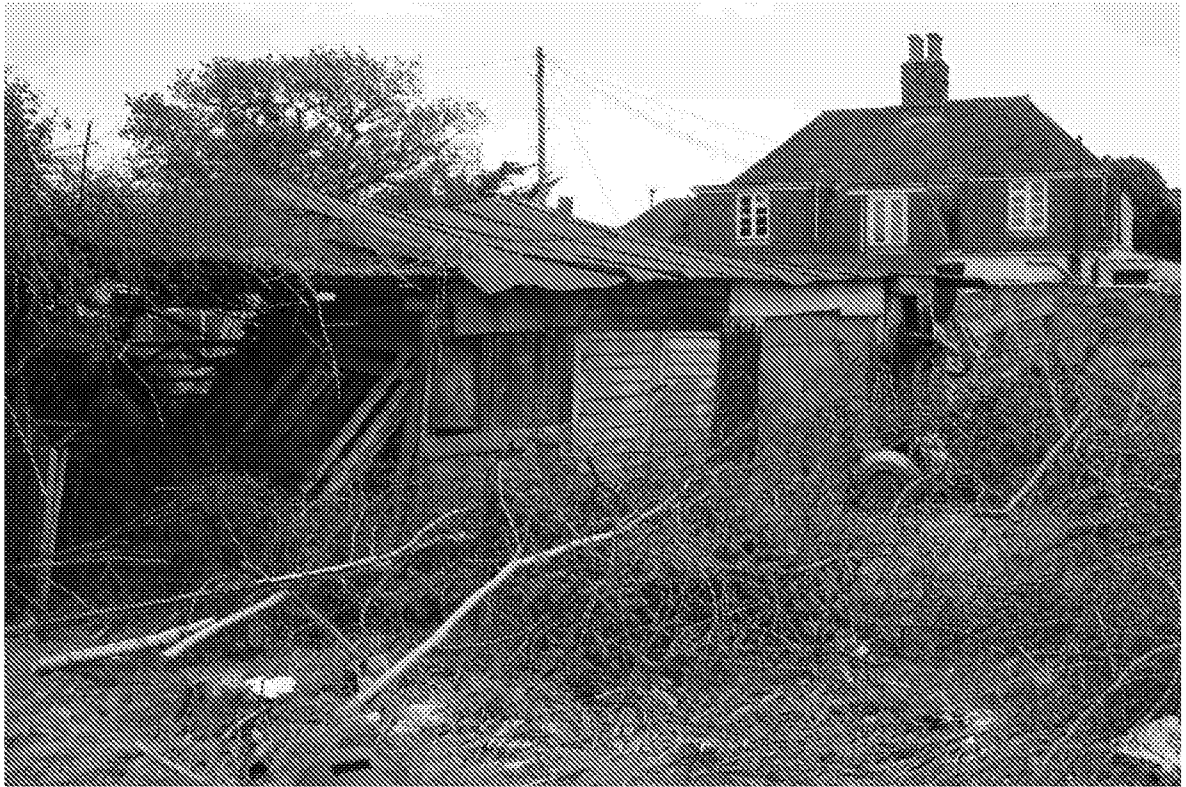
Derelict buildings at south-east end of site
