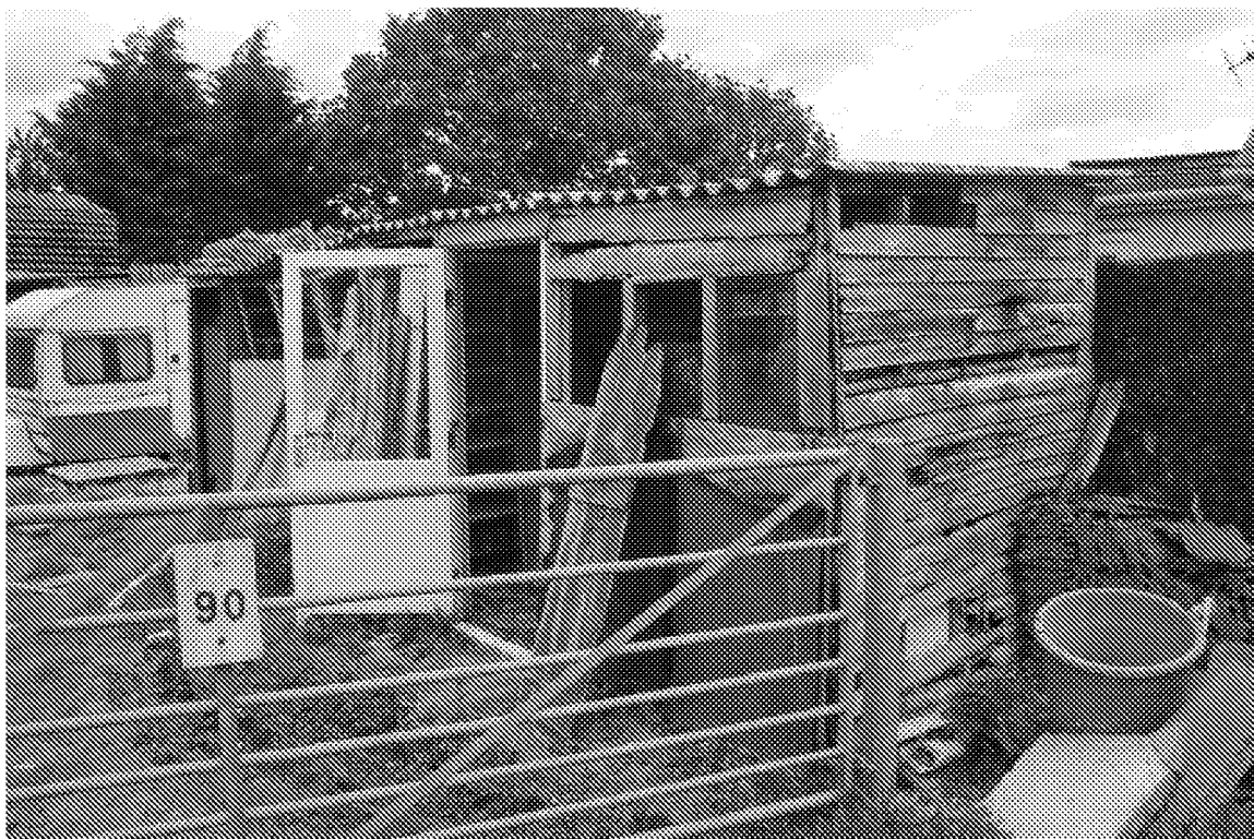
Access gate and derelict buildings at south-eastern end of site
