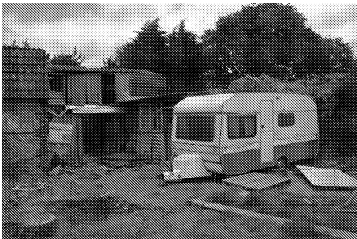
Derelict buildings and caravan at north-east end of site
