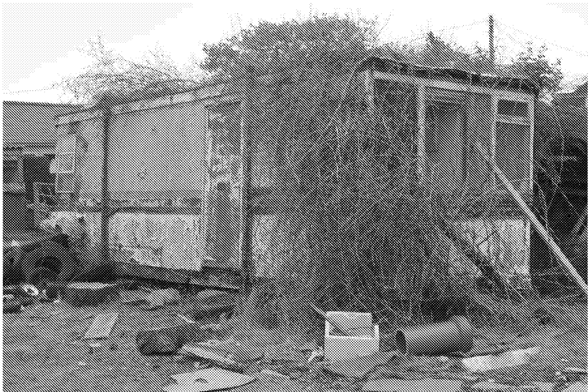
Derelict portacabin in centre of site
