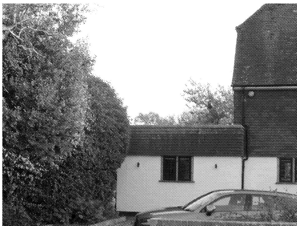
3 – Area to be demolished and replaced
