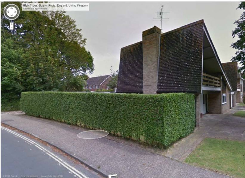
Road View Including Existing House
