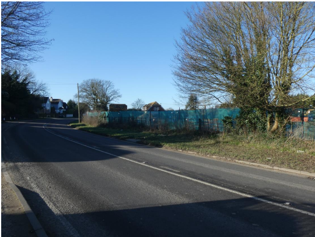
SECURITY FENCE FONTWELL AVENUE
