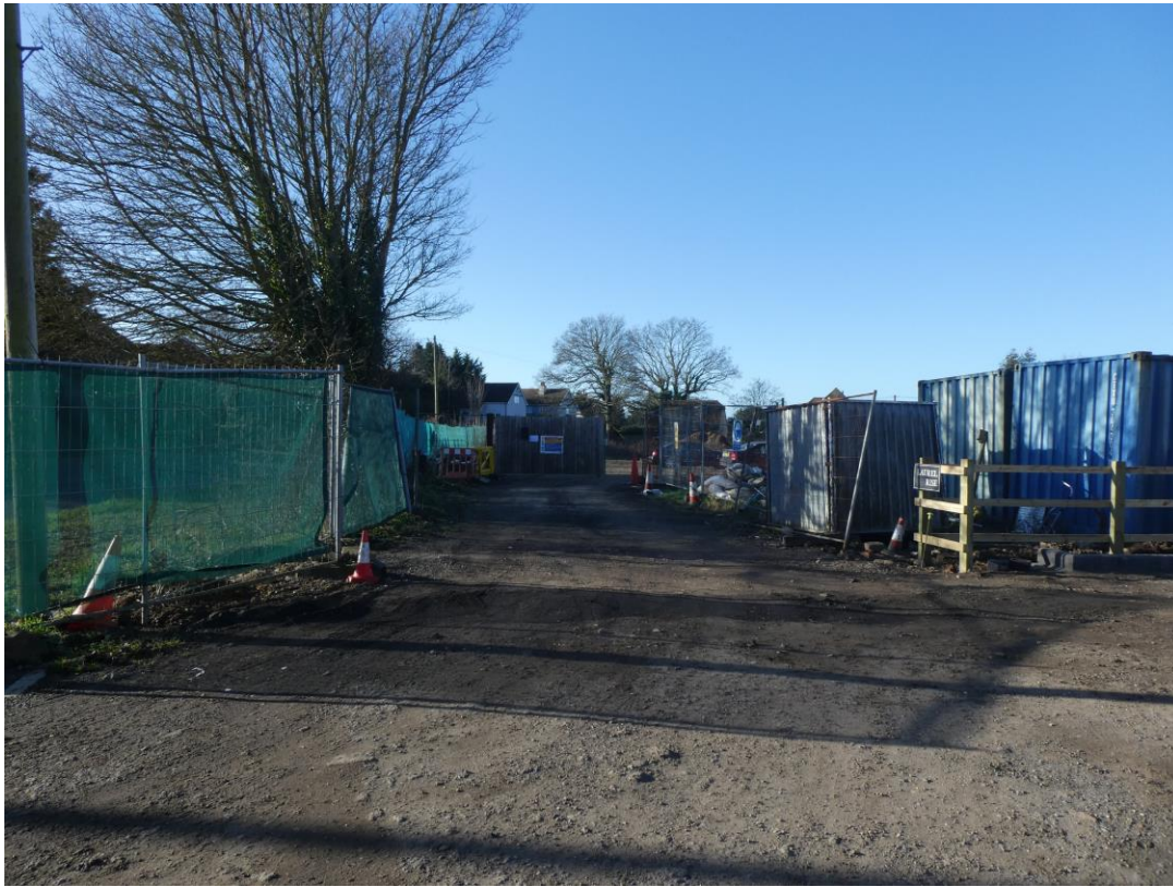
GATE ENTRANCE TO SITE
