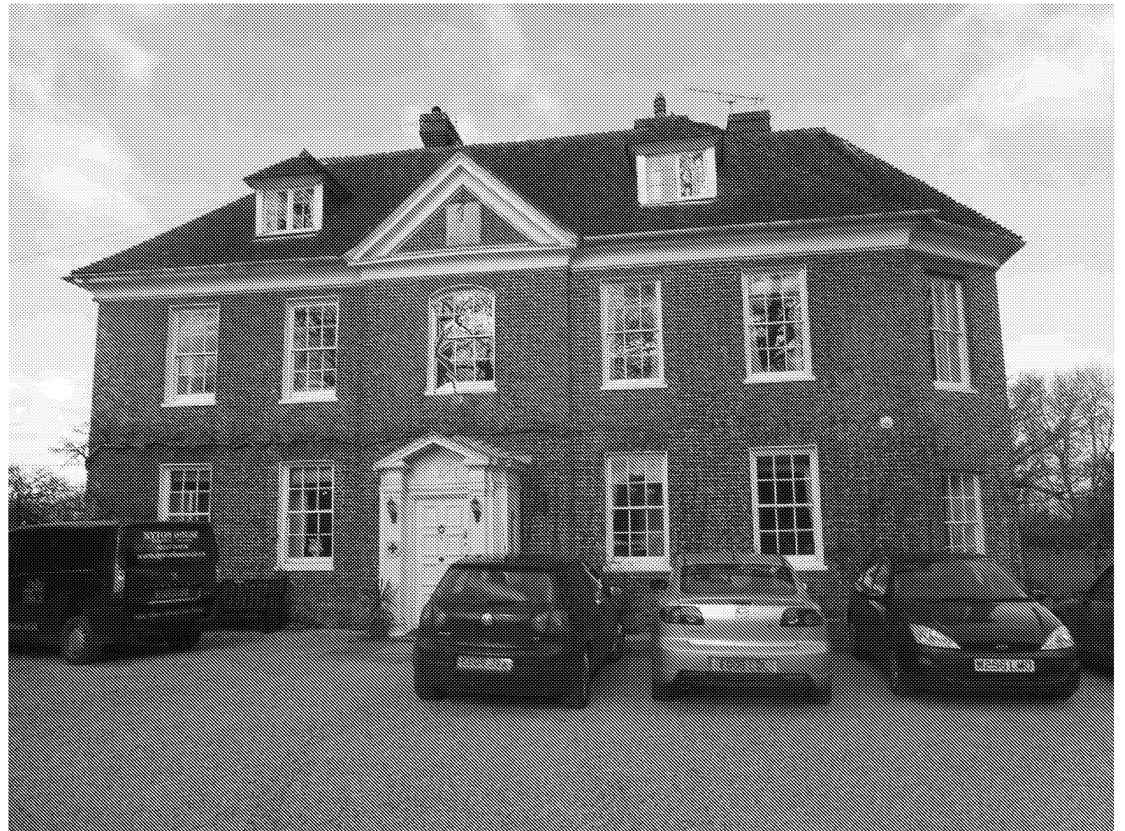
03: Main entrance of Nyton House (South Elevation)
