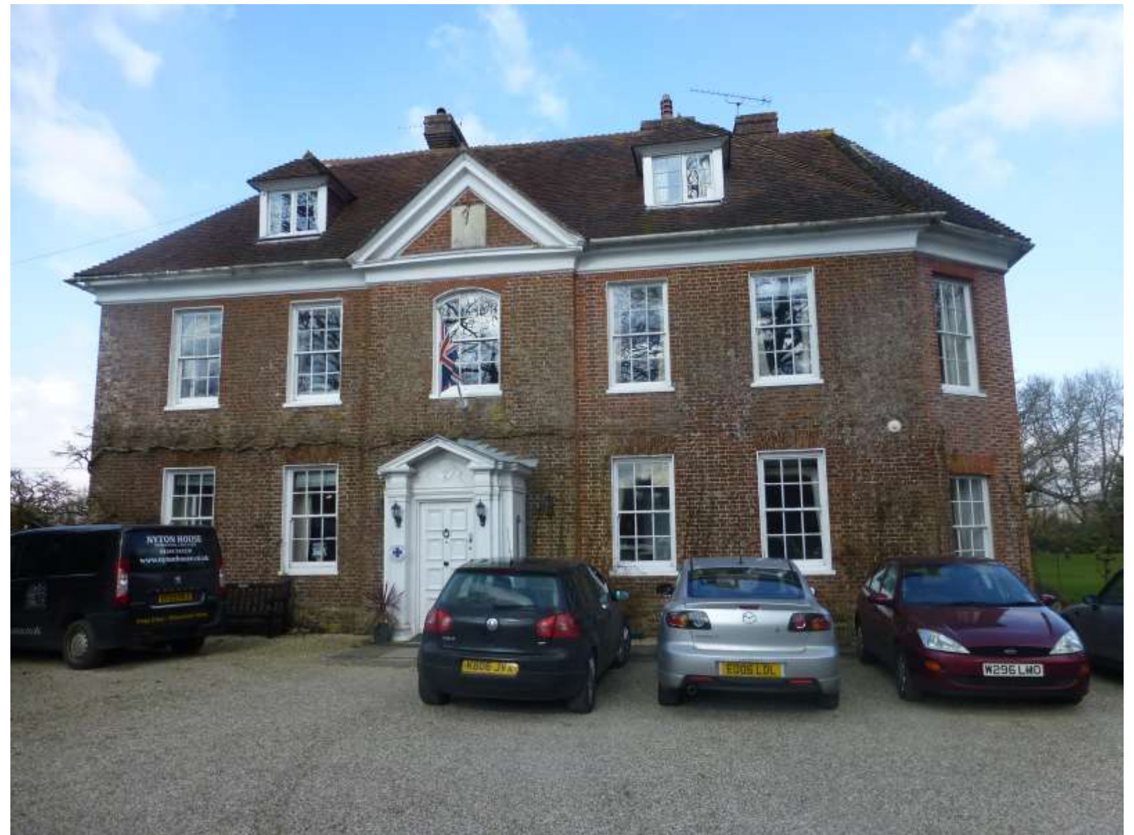
03| Main entrance of Nyton House (South Elevation)
