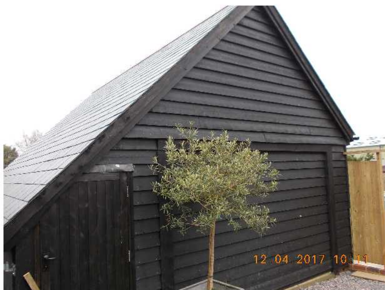
Kitchen (Carport) north elevation
