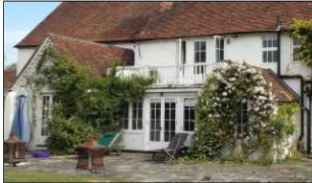
The single-storey extension on the south side of the house, looking north.
