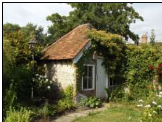
The potting shed, from the north-east.
