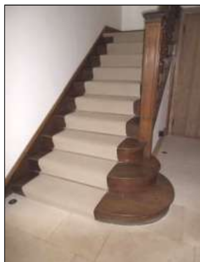
The staircase, looking south.
