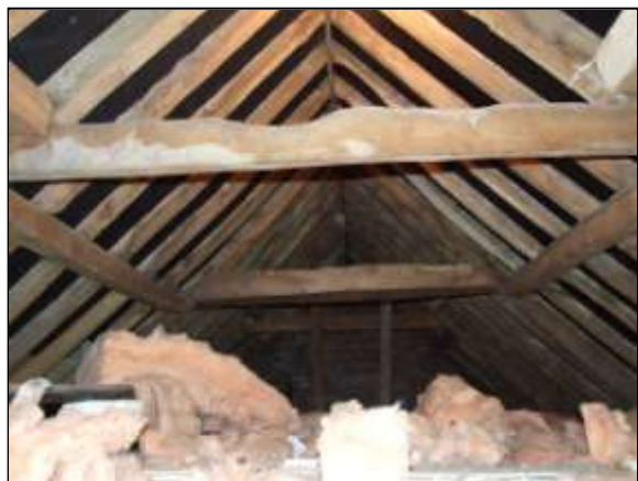
The roof, looking west.
