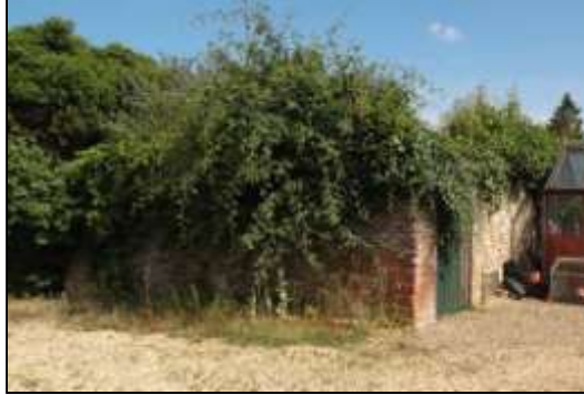
The farmyard wall, looking north.
