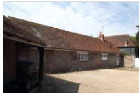
Stable Cottage, from the north-east.
