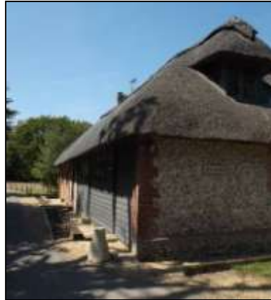
The Barn, from the north-east.
