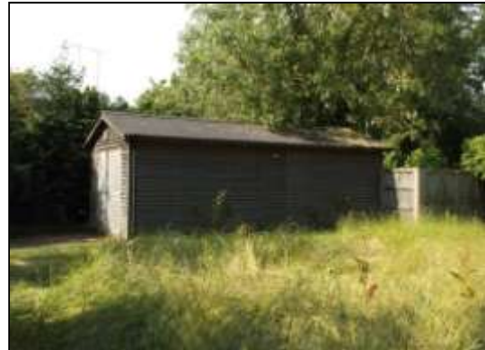
The garage, looking south.
