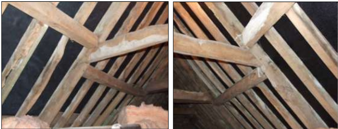
The two ends of one of the trusses in the roof, looking east.
