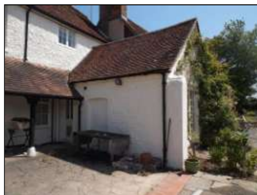
The Phase 4 addition, from the west.
