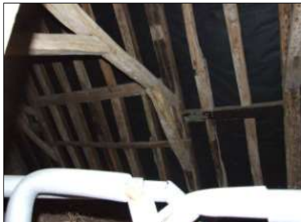
Part of the roof frame, looking south-east.
