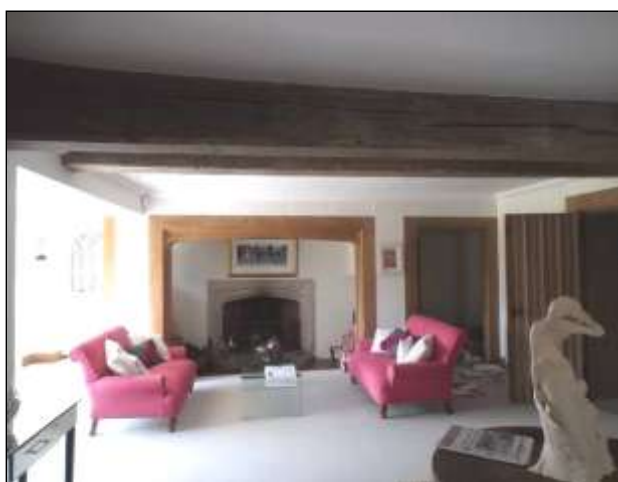
The ground floor of the house, looking west towards the possible inglenook fireplace and with the two cross beams in the foreground.
