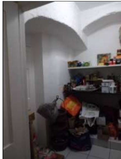
The larder, looking south.
