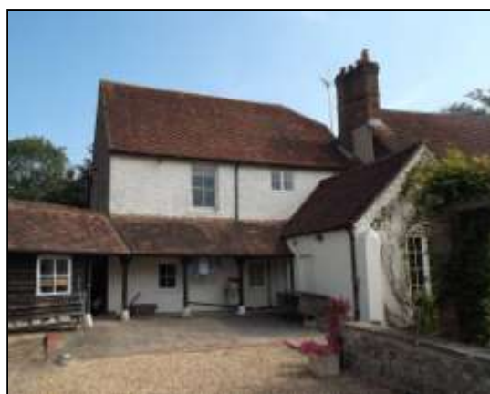
The house from the south-west.
