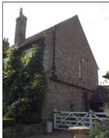
The west elevation of the Phase 3 extension, looking south-east.
