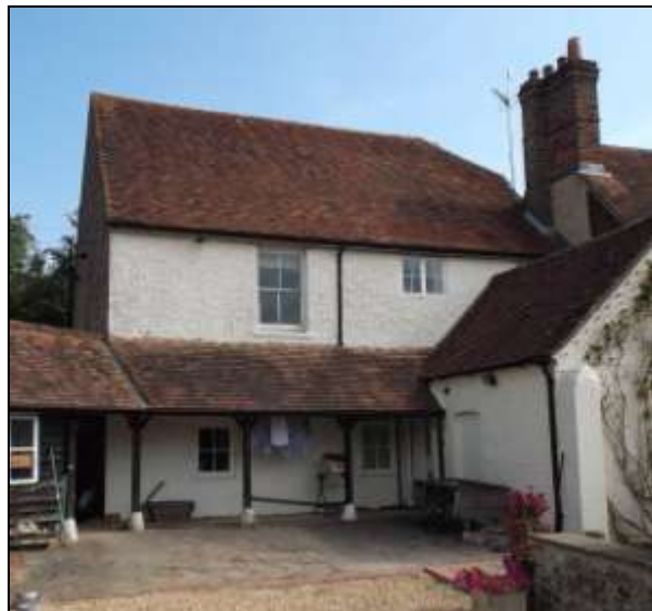
The south elevation of the Phase 3 extension, looking north.
