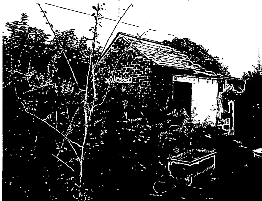
Rear Elevation of Detached Building
