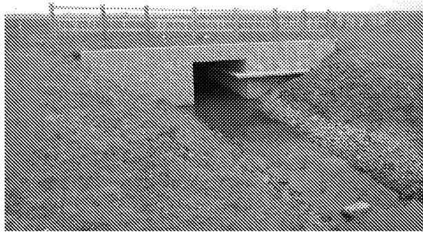
Figure 2- Culvert with Ledges for Mammal Passage
