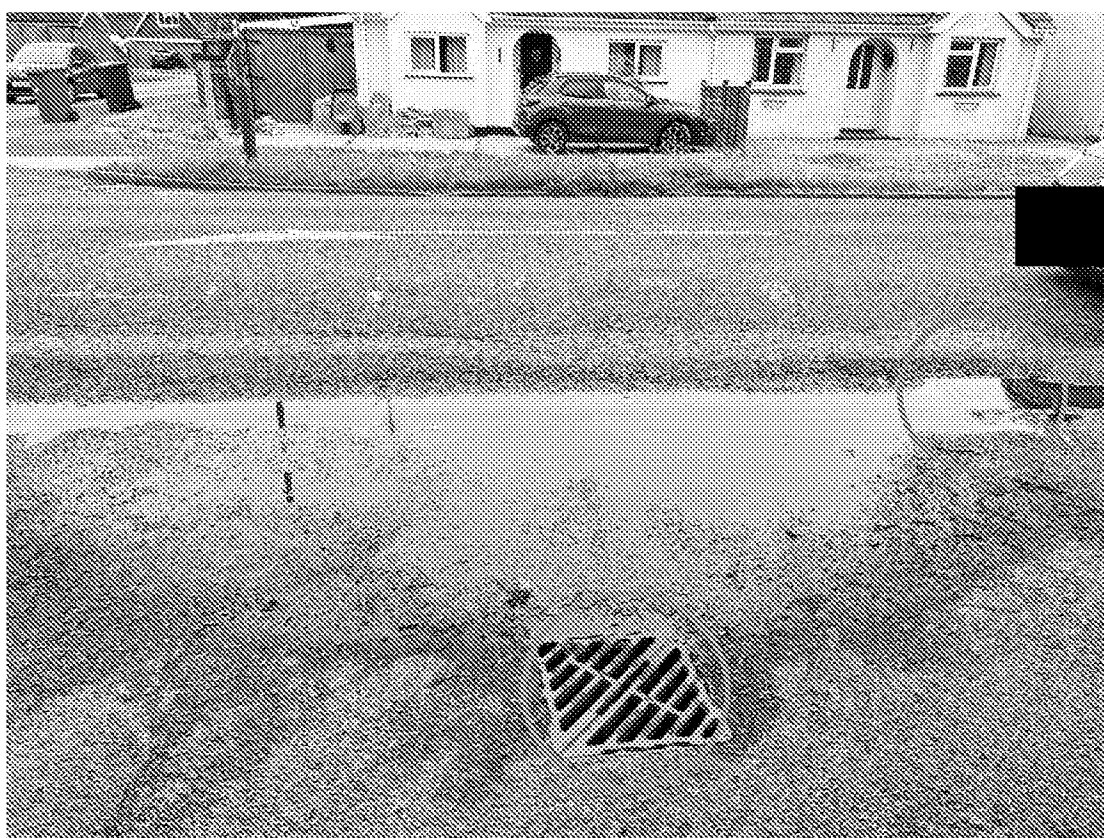
View from footway/cycleway link onto proposed cycle crossing location
