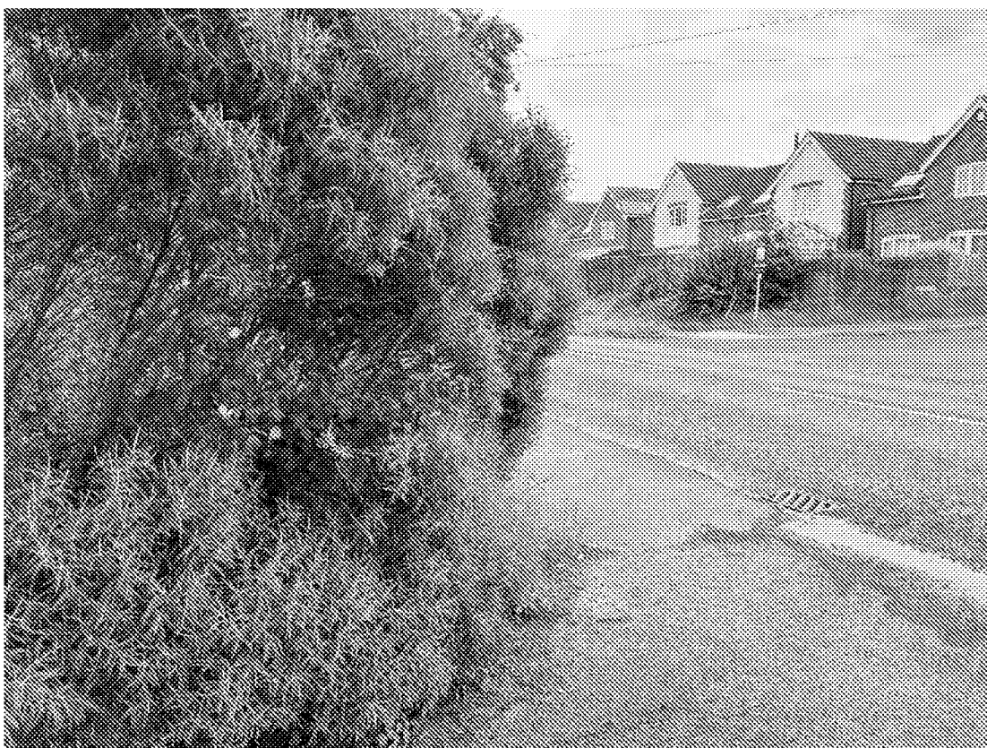
View looking north west from proposed footway/cycleway link impeded by vegetation
