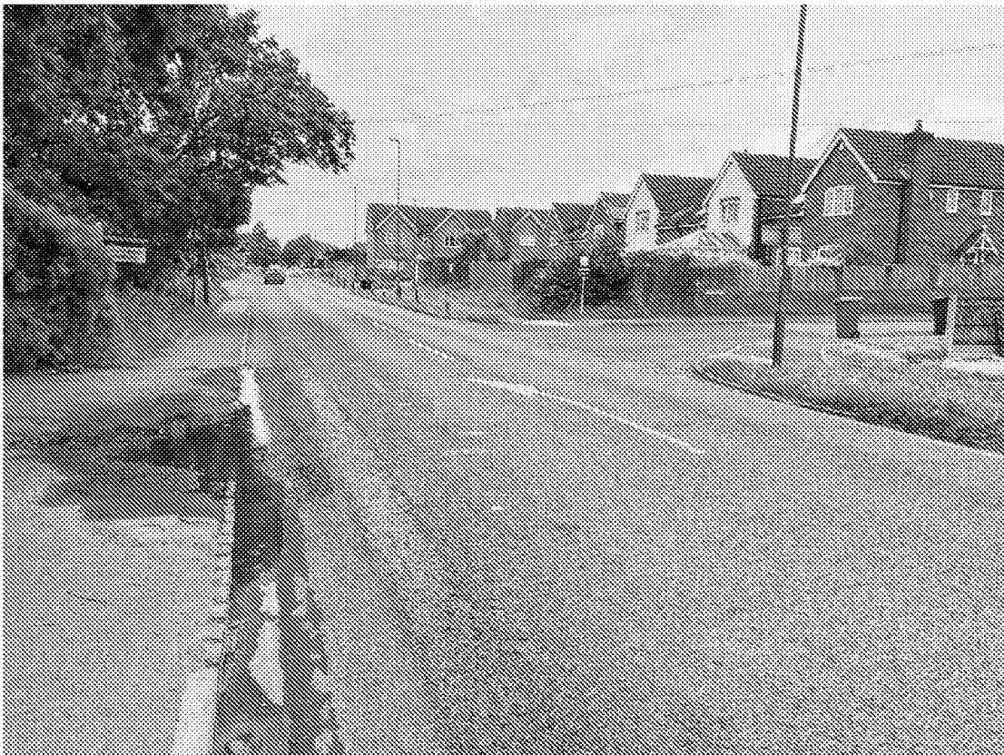
Looking north on Lidsey Road at the proposed cycle crossing site. Note level crossing in background
