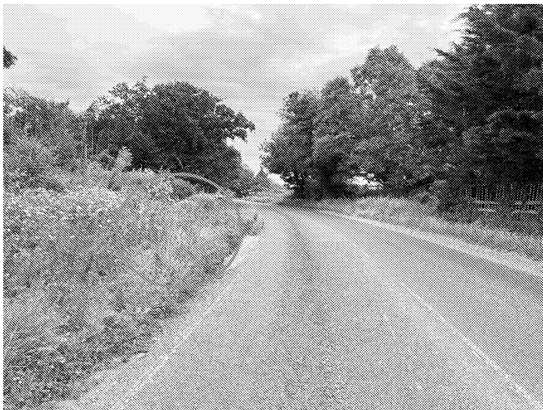
View of Lidsey Road in a northerly direction, at location of proposed local road widening, new access formation and right-turn lane
