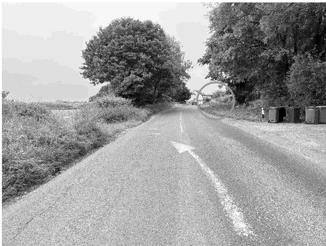
View of Lidsey Road in a southerly direction (proposed main vehicle access within the verge to the right)
