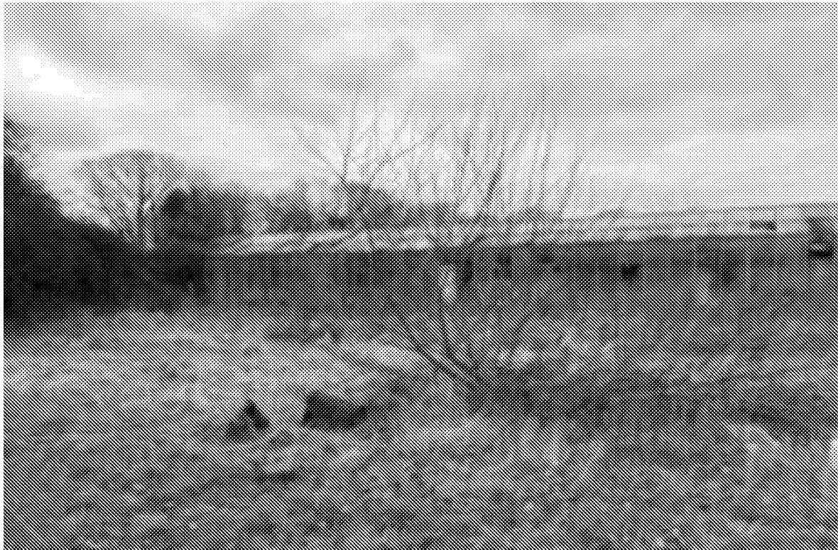
A current view of the proposal site at Woodgate Nurseries, including its redundant buildings
