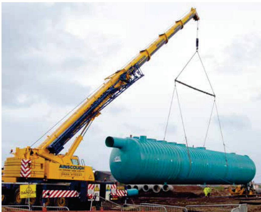
SPEL Puraceptor Class 1 full retention single chamber separator NS942 with 'automatic' Econoskim System serving a large catchment area (5.0 hectares) at Bristol International Airport.
