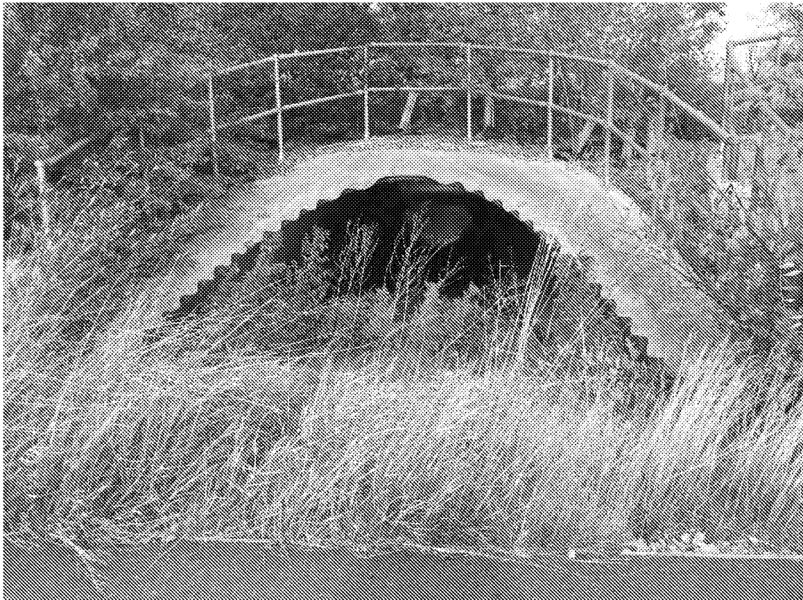
Flood Tunnels (approx. 1.2 m to 1.5 m Ø)
