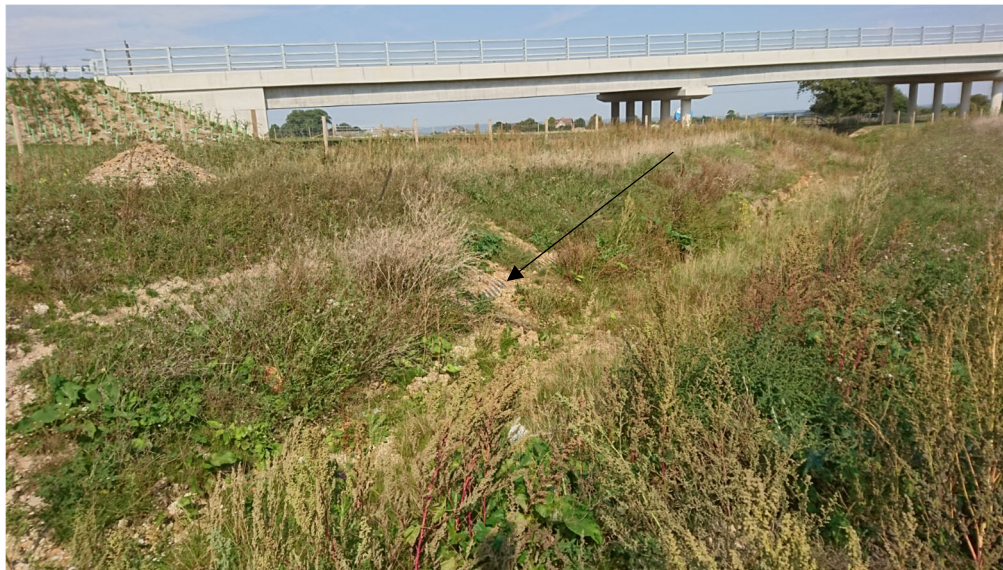
Figure 2: Photograph of site showing existing corrugated pipe – assumed land drain.
