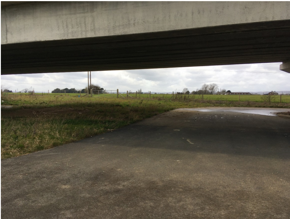
Photograph 1 –View beneath flyover looking north east
