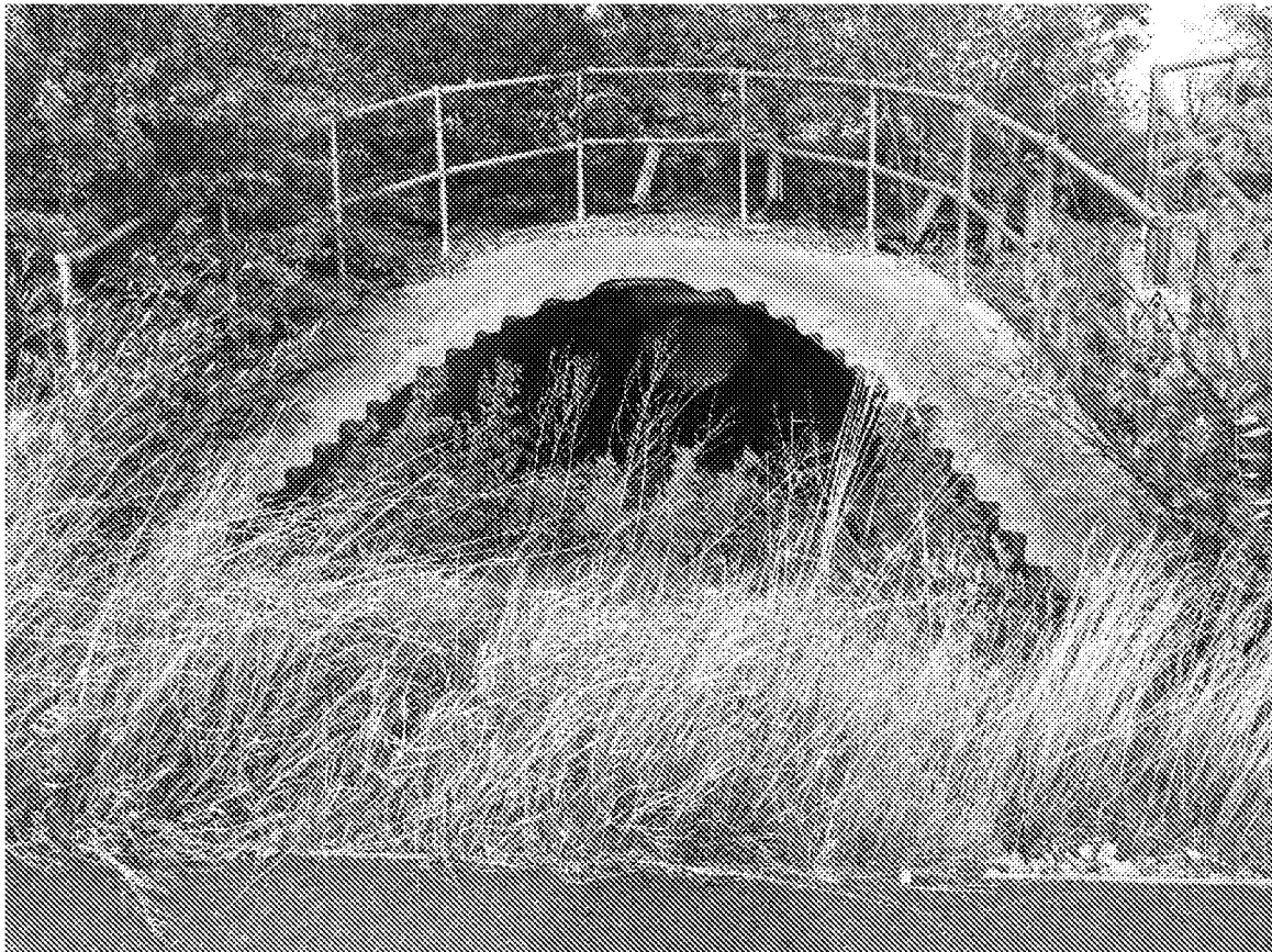
Flood Tunnels (approx. 1.2 m to 1.5 m Ø)
