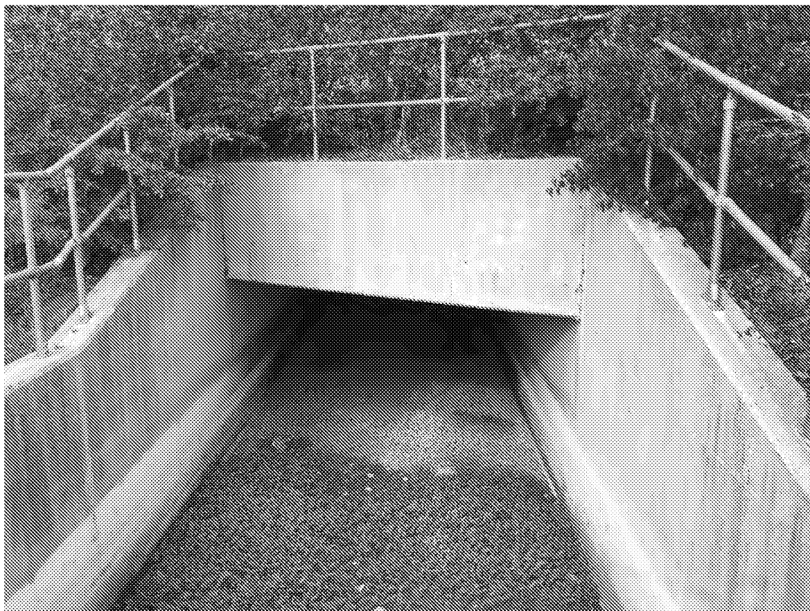
Oldland Farm Ditch A259 Culvert (approx. 4.0 m x 2.5 m)
