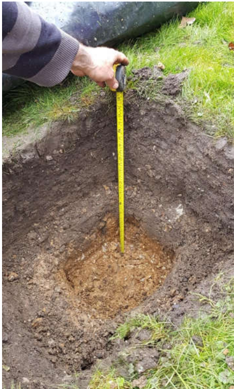
Excavated hole with 300mm square base
