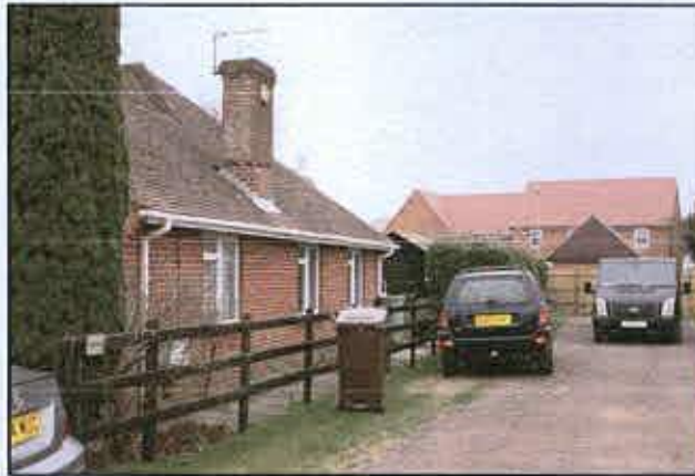
Side view of bungalow looking south
