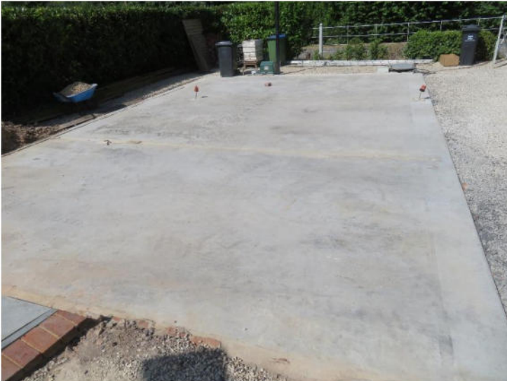
IMG 1436 Overall view of the triple bay garage
