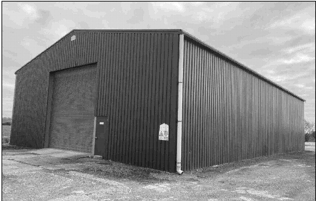
Photograph 4. Building C viewed from the south-west.
