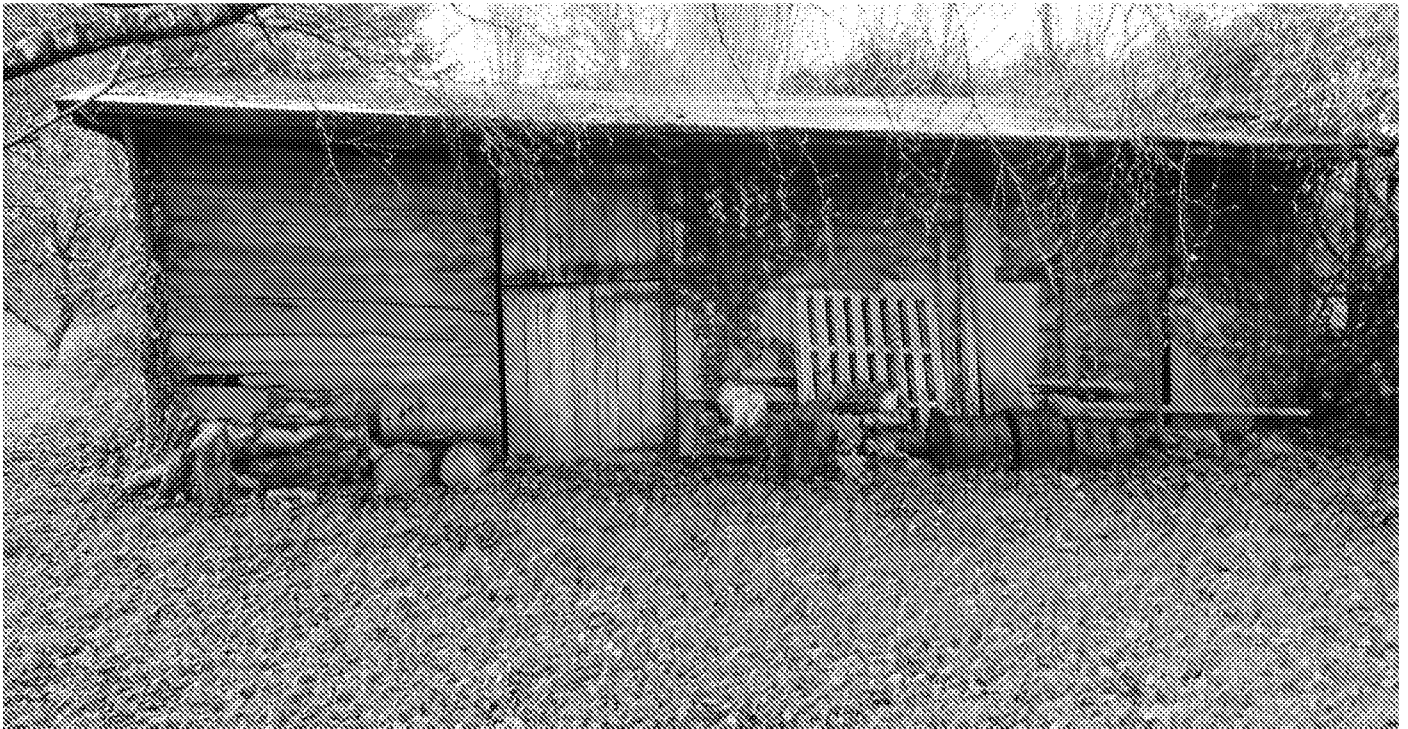
Photograph No. 7 - Building B4, assessed as providing 'negligible' bat roost suitability.
