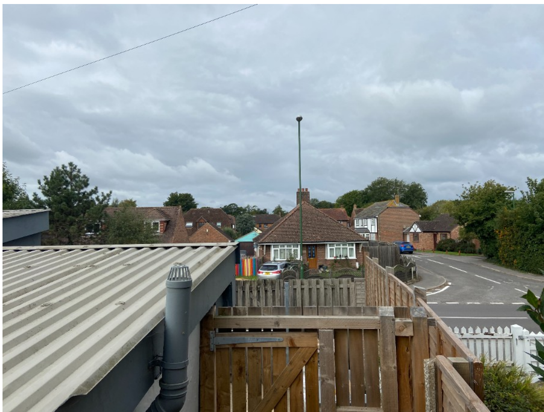
View from HGC North East corner over boundary fence showing road view and current workshop roof structure. This ground level is approx 2.5m above the street level.
