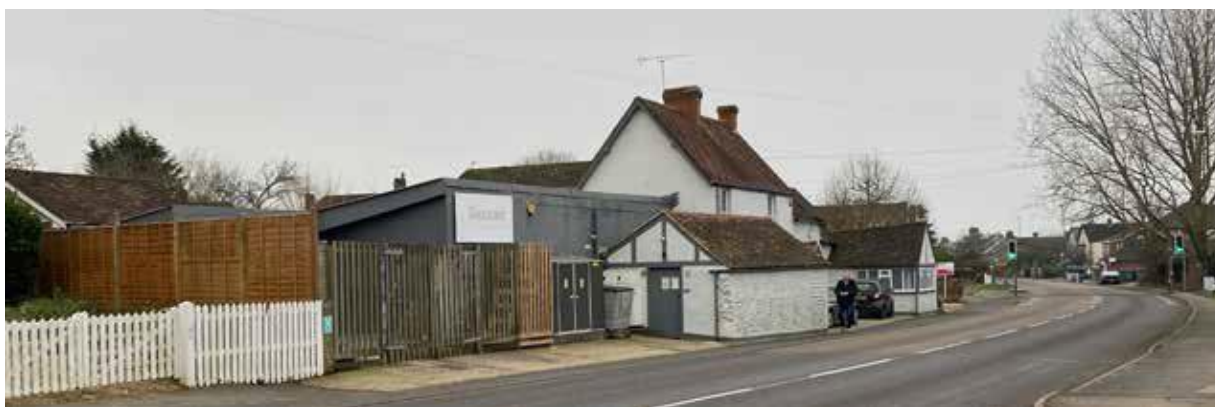
Existing garage on boundary with footpath
