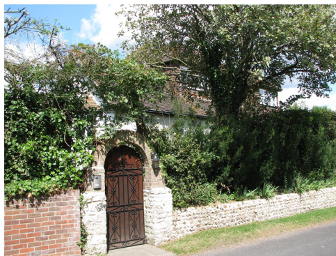
2195 - Pedestrian Gated Entrance: Flint & brick walls; Black Iron Gate with solid timber infill behind; Mature hedges.
