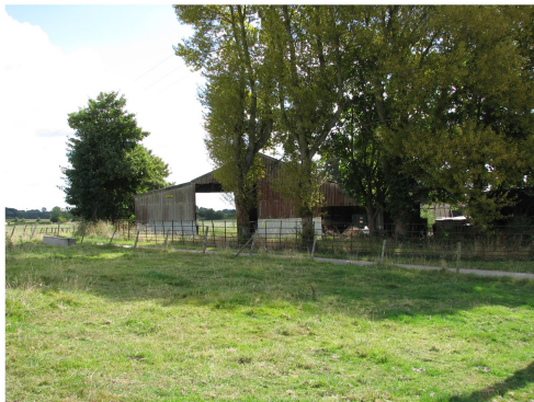
2177 - Half Timbered Barn: Vertical timber cladding.
