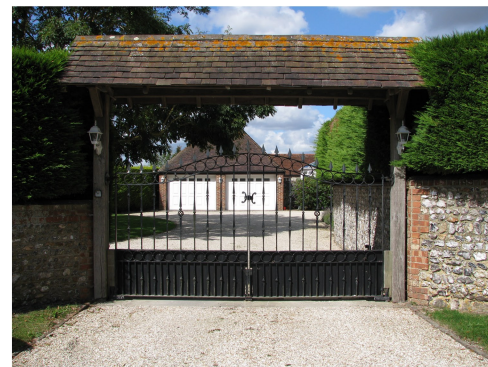
2172 - Gated Entrance: Black Iron Gates; Flint wall with brick piers and quoining; Gravel courtyard.
