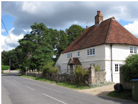
2246 - Rose Garden Cottage: Cat slide roof; Shallow front garden; Flint wall with brick piers and flint infill - no quoining.
