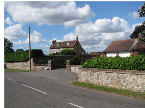
2163 - Boundary Treatment: Flint walls with brick quoining; Mature hedges.
