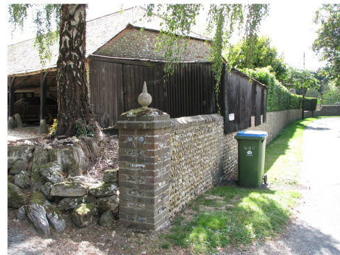
2120 - Timber Frame Barn: Single storey; Long & thin; Infill flint walls with brick quoining; Open fronted; Slate roof; Gravel Courtyard.
