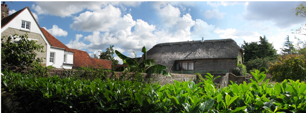
2135 - Thatched Dwelling: Flint gable walls with brick quoining; Timber clad long elevations; Thatched roof; Dark windows.
