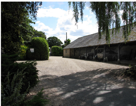
2120 - Timber Frame Barn: Single storey; Long & thin; Infill flint walls with brick quoining; Open fronted; Slate roof; Gravel Courtyard.
