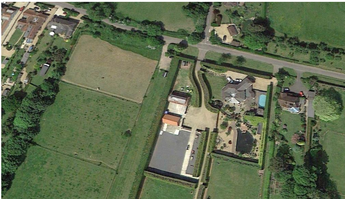
Figure 3 – Aerial photograph of application site
