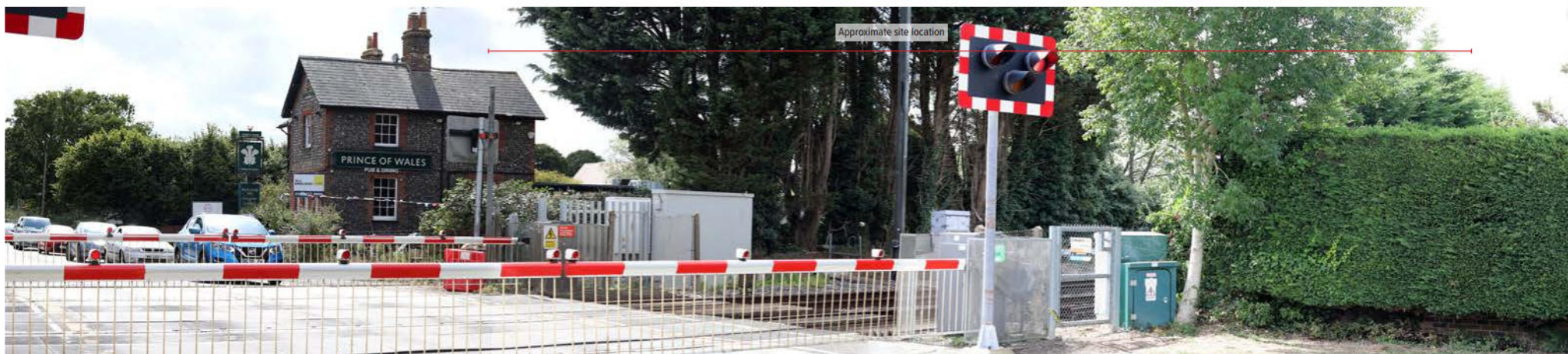
RVP 03 - View southwest from Lidsey Road junction with level crossing
