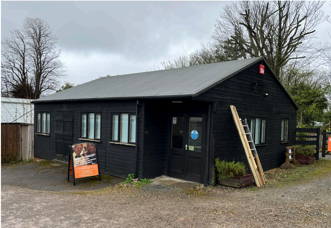
Photo 1 – Existing Building (north elevation)
