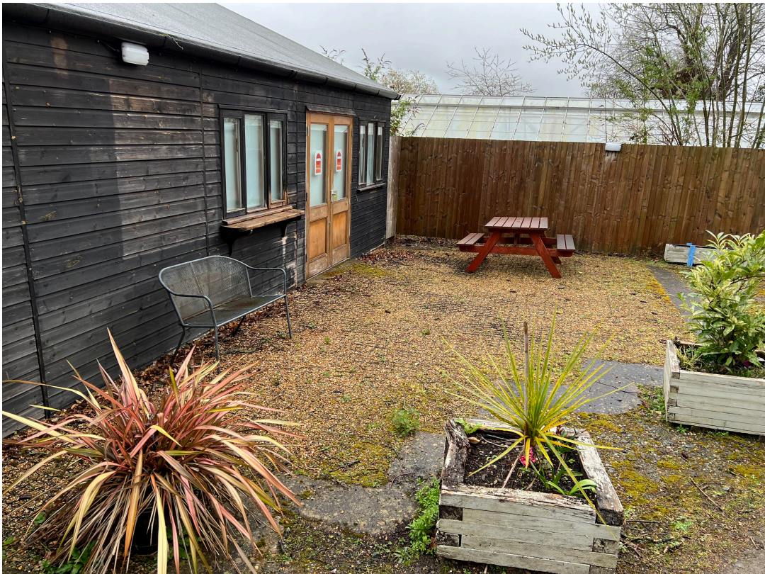
Photo 2 – Existing Building (south elevation)
