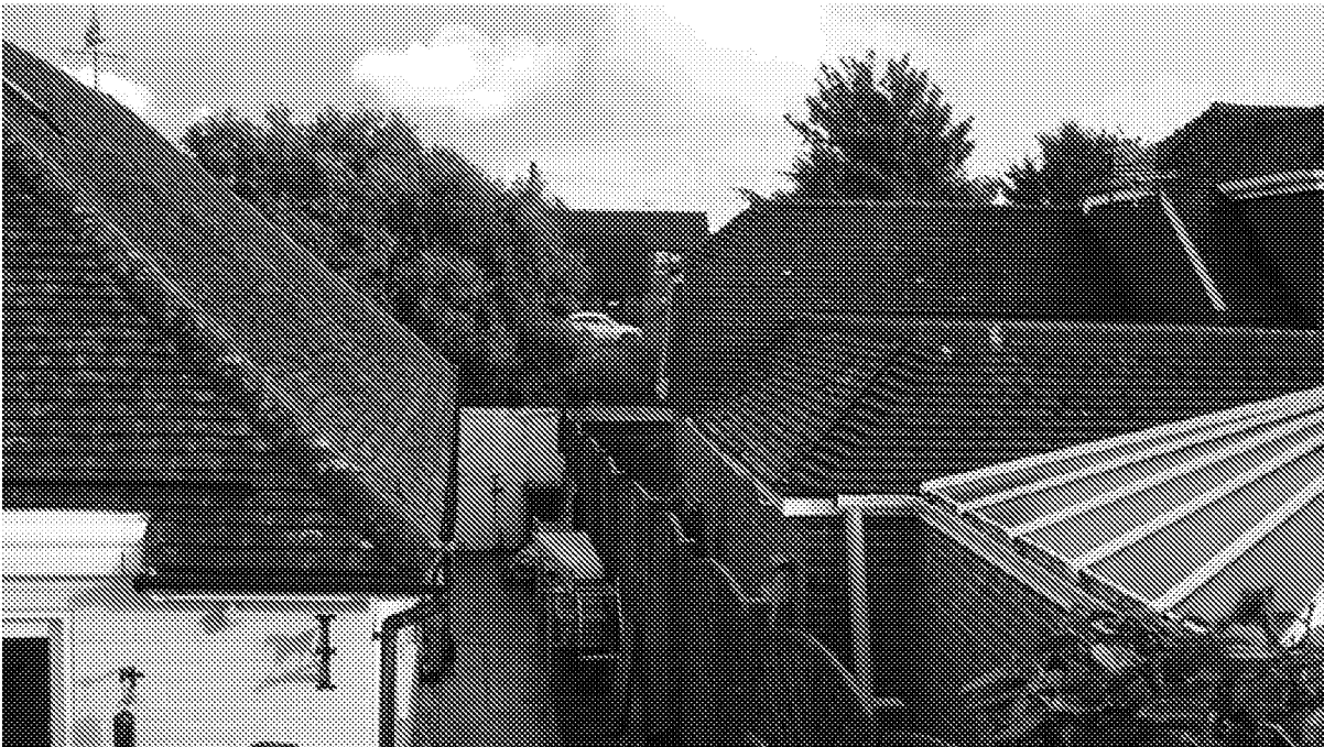
Elevated side view showing roof line which will be extended.
