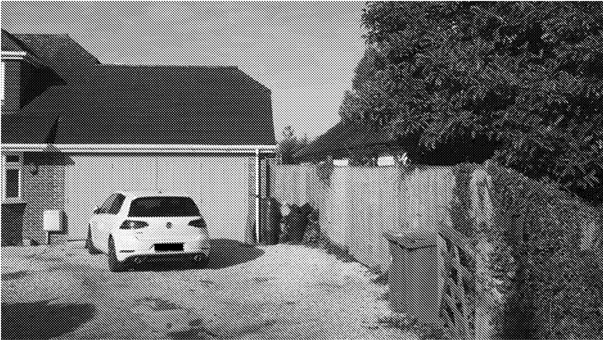
Present front view showing proximity to the boundary.
