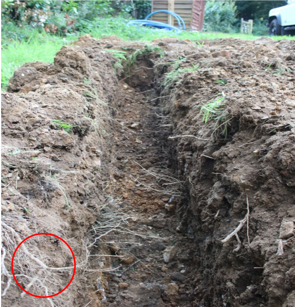
Fig. 5 – excavation within raised ground; note grass roots at all levels and <10mm Ø laurel root circled.
