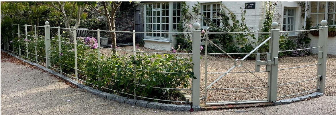
Fence and pedestrian access gate (Height -
