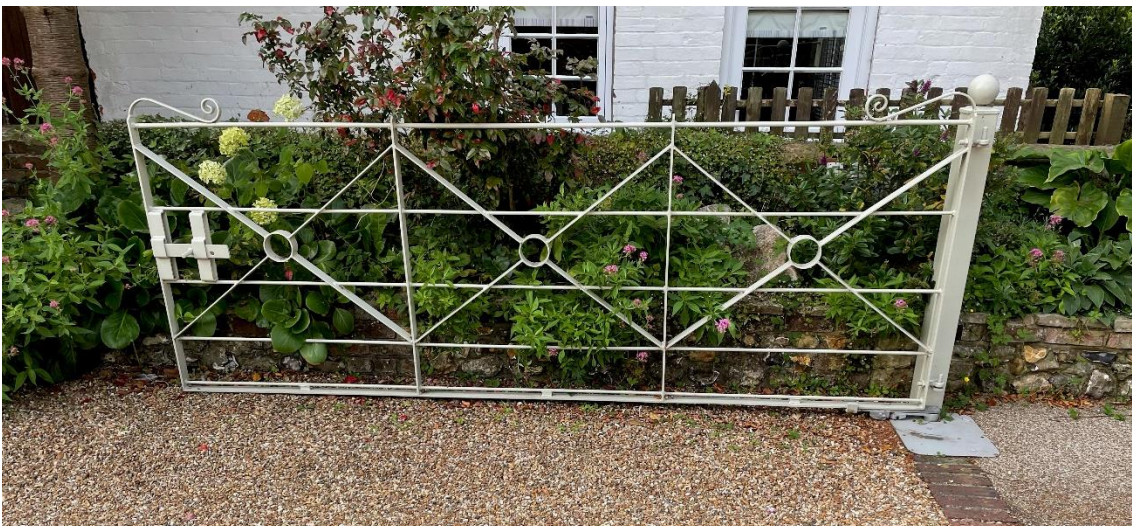
Vehicle Access Gate
