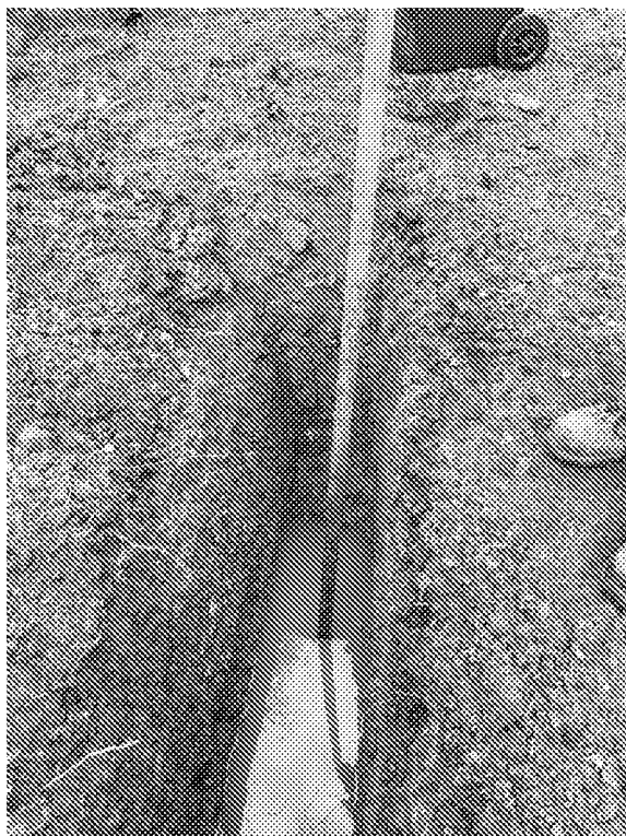
Soakaway Test excavation hole
